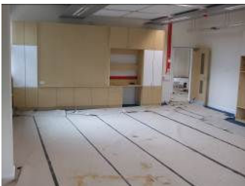
First floor Classroom 4G fitted furniture typical progress.
