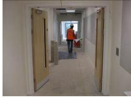
Ground floor circulation C4/C5 viewed north progress.
