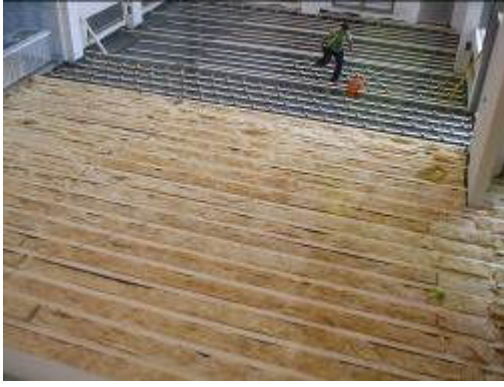
Hall/Dance studio floor progress viewed from above.
