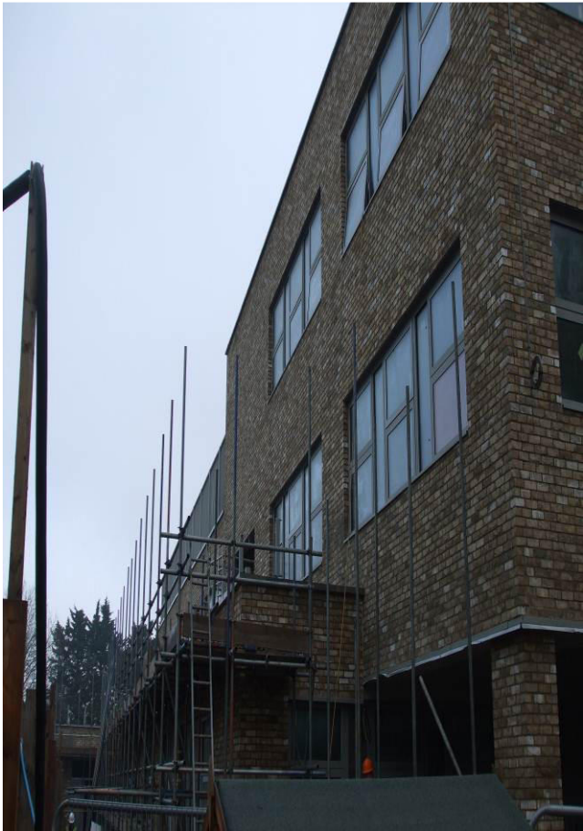
Photo 1 - Rear elevation viewed from Main Gate.
