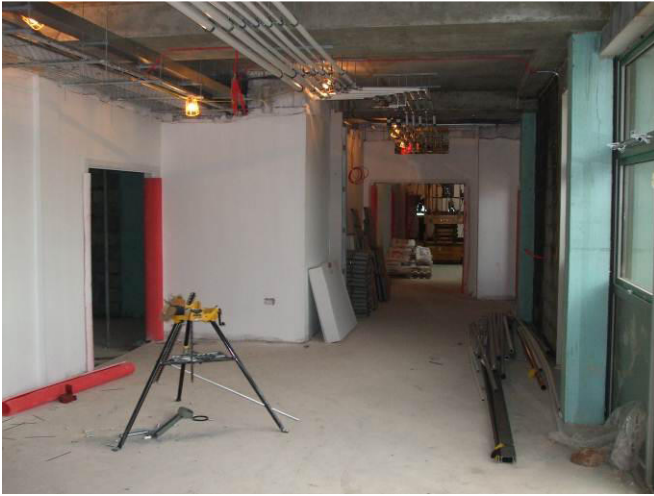
Photo 5 - Ground floor viewed from north adjacent to the WC.
