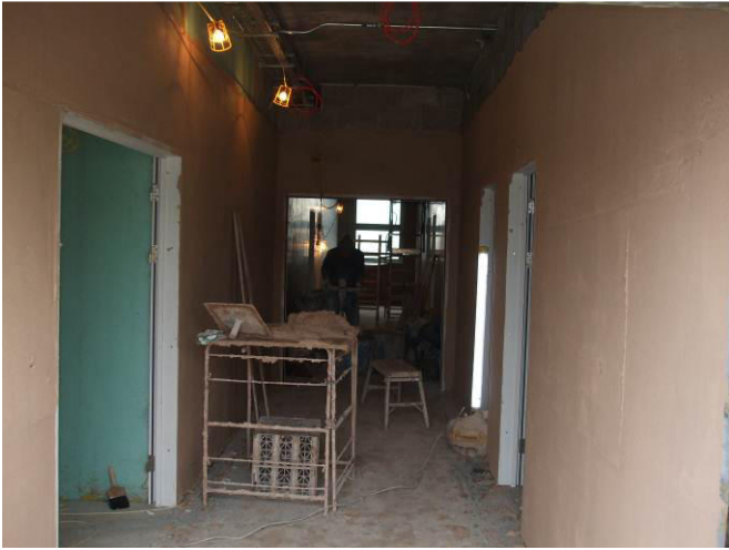
Photo 11 - South tower progress viewed from the roof access doors.
