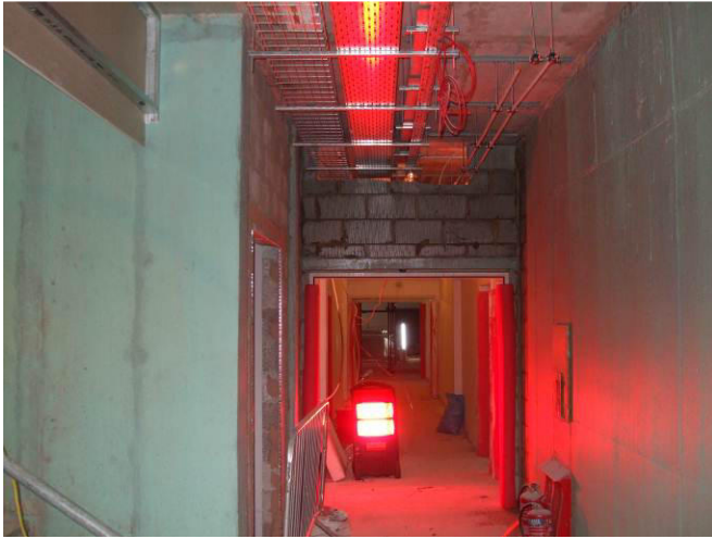
Photo 4 – Ground floor viewed south from north end door.
