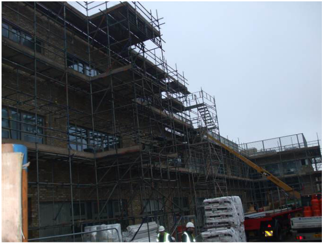
Photo 2 - Front elevation viewed from south end of side.
