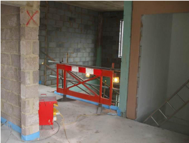
Photo 9 - North tower progress viewed from the roof access doors.
