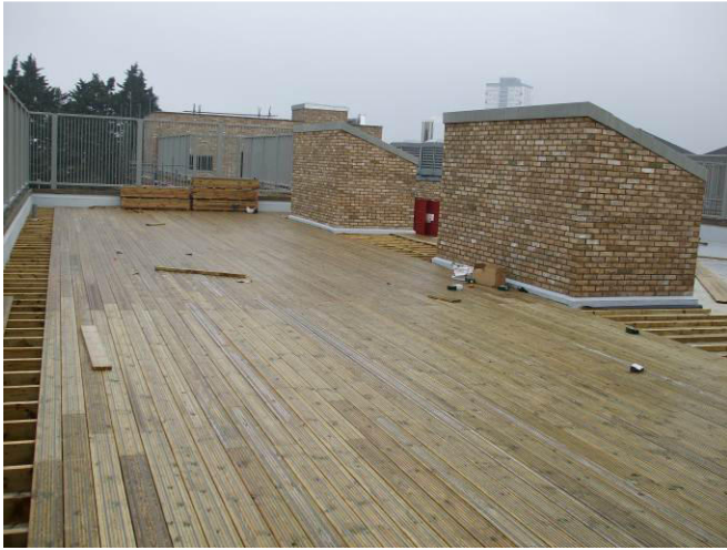
Photo 10 - Roof terrace (decked teaching area progress).
