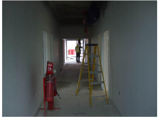
Photo 2 – Internal second floor circulation area progress.
