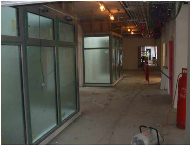
Photo 9 – Internal first floor circulation area showing light well 1 and 2 progress.
