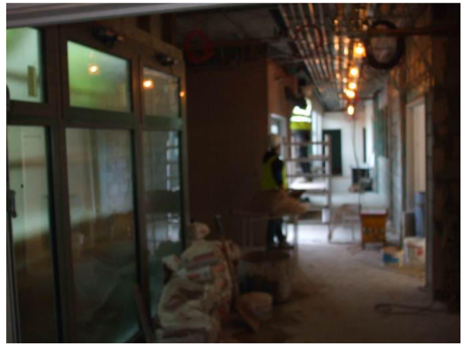
Photo 10 – Internal first floor circulation area showing light well 3.
