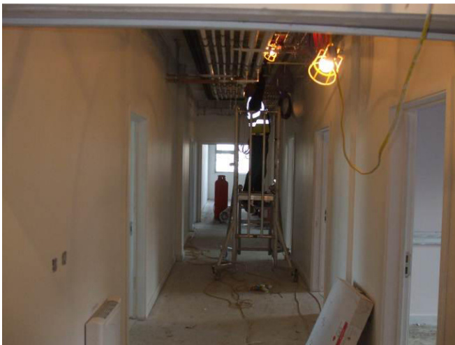
Photo 11 – Internal first floor circulation area viewed towards north end.
