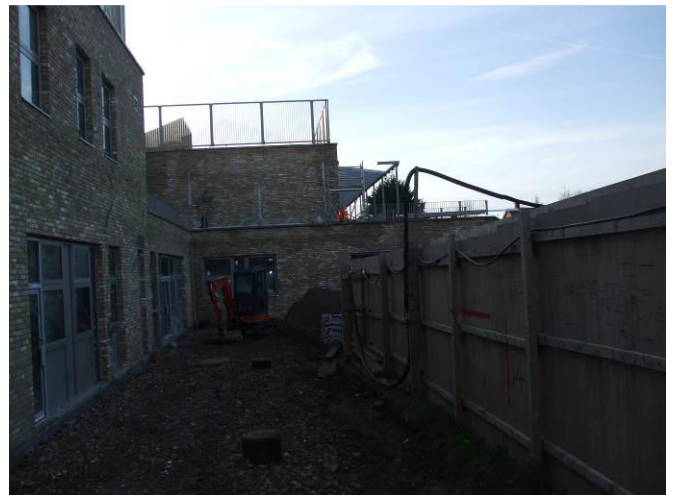
Photo 12 – External rear elevation showing glassed canopy to walkway.
