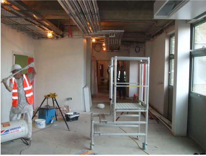
Photo 14 – Internal ground floor circulation area.
