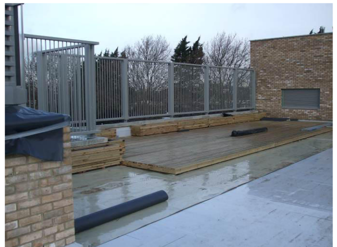
Photo 6 – External roof terrace left side viewed north.
