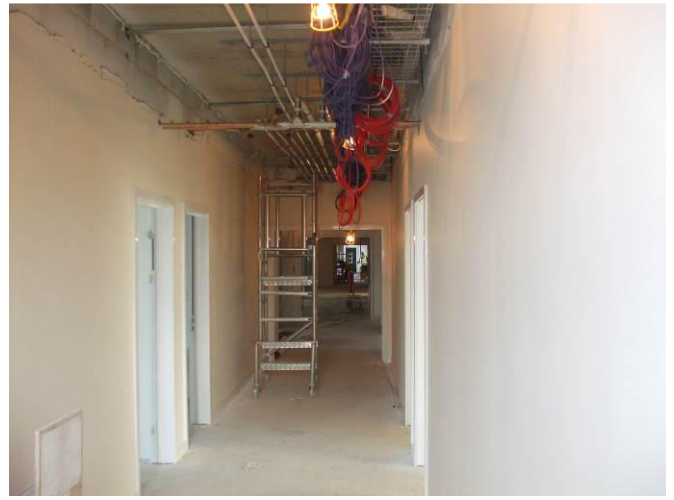
Photo 8 – Internal first floor circulation area viewed north.
