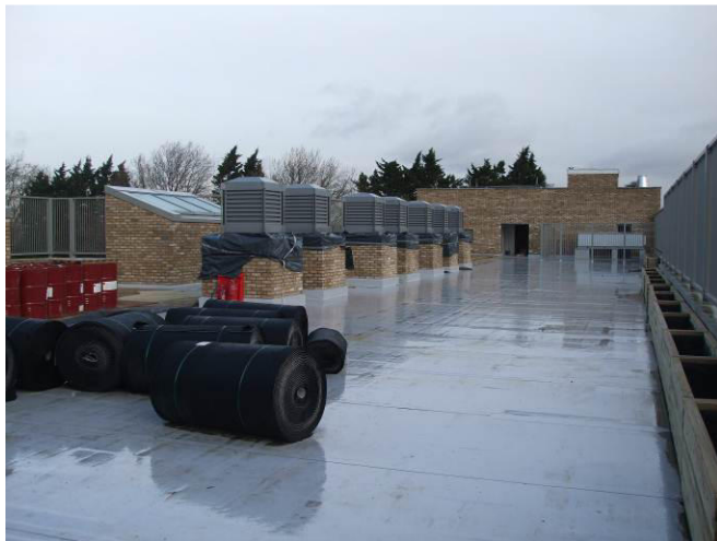
Photo 3 – External roof terrace viewed from south looking north left side.
