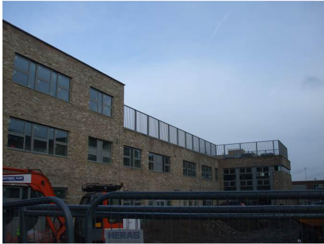
Photo 1 – External front elevation.
