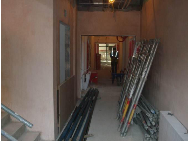
Photo 13 – Internal ground floor circulation area.
