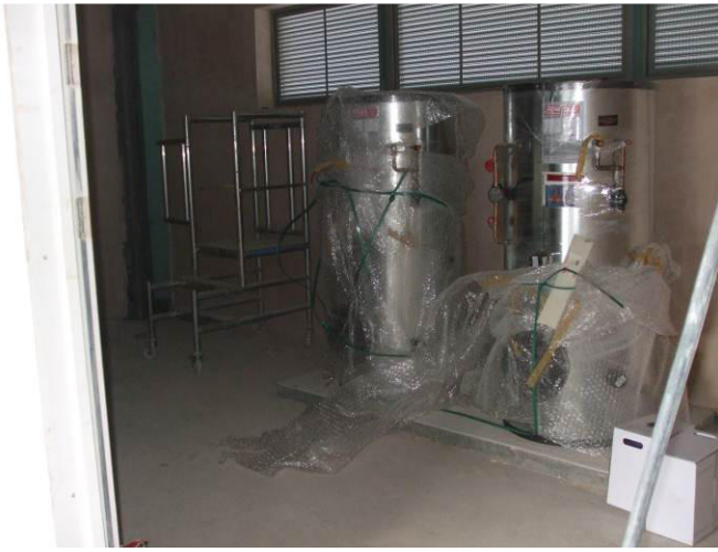
Photo 7 –Internal plant room progress.
