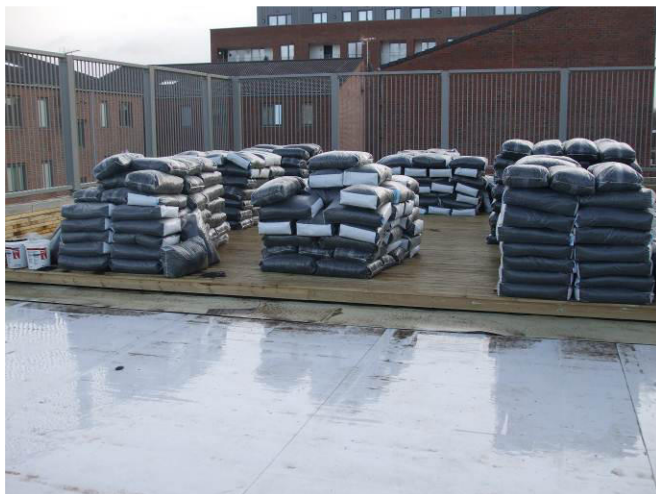
Photo 5 – External roof terrace front right looking north.
