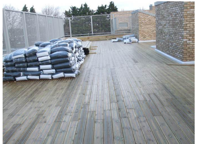
Photo 4 – External roof terrace decked teaching area viewed north.
