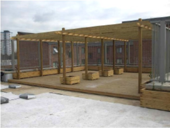
Photo 1 Pergola in progress - Roof
