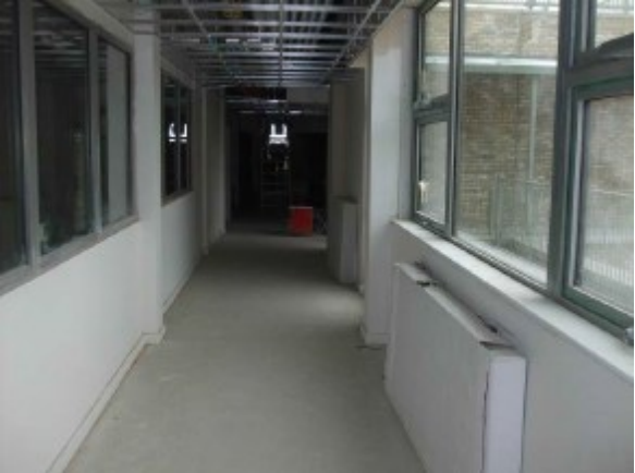
Photo 2 First floor corridor
