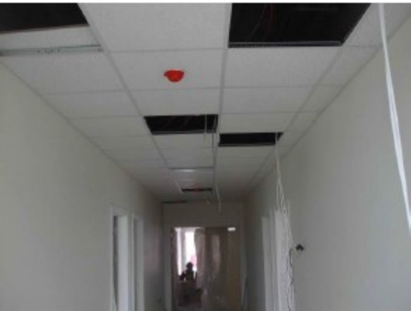
Photo 3 – 2 nd floor ceiling in progress
